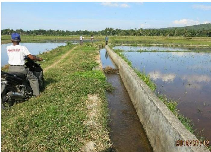
**Irrigation canal in Manyang Lancok village with incomplete design and lack of maintenance.** The canal is missing field gates. The community is not performing basic maintenance such as cleaning overgrowth. (World Bank, 2018)
